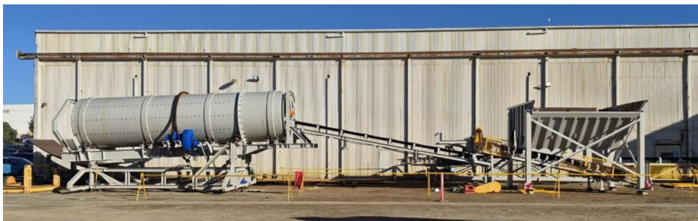
Figure 10: OZM feed bin, feed conveyor and agglomerator drum at Polaris Engineering Services Henderson Facility
