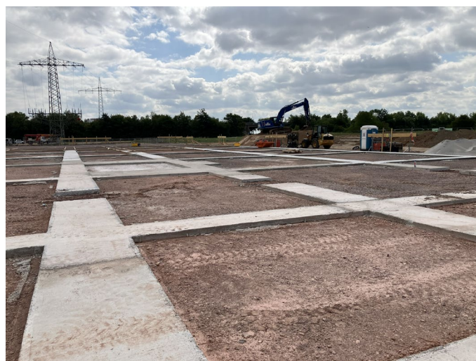
Figures 3 & 4: First concrete layers for the Lionheart geothermal power plant in Landau which will act as a base for foundations
