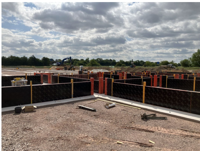
Figures 3 & 4: First concrete layers for the Lionheart geothermal power plant in Landau which will act as a base for foundations
