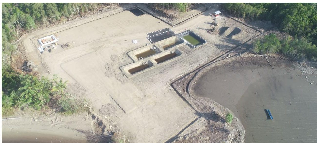
Figure 1: Bula Karang well location with site construction near completion (photo taken mid-July 2026)
