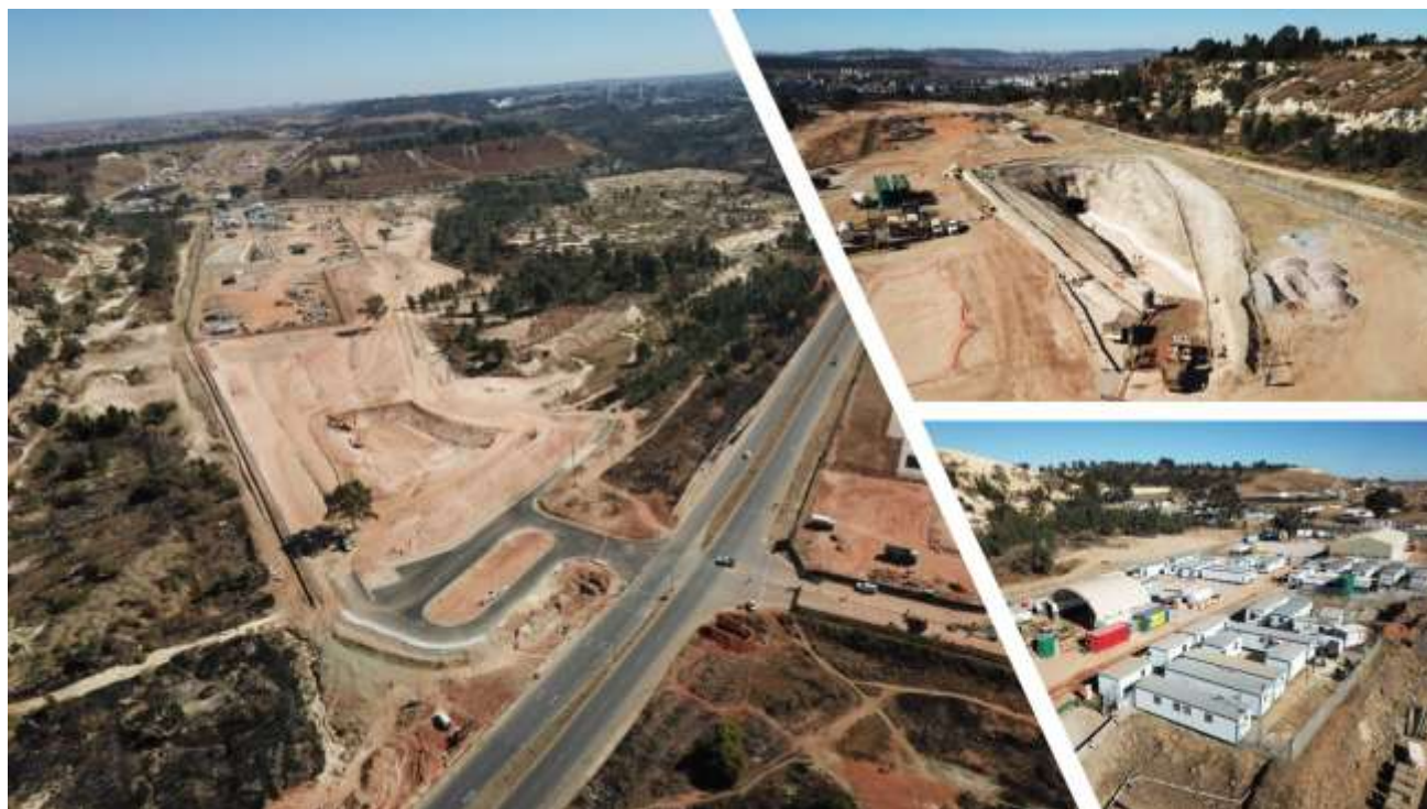
IMAGE 1: AERIAL VIEW OF QALA SHALLOWS WITH DEVELOPMENT OF SURFACE INFRASTRUCTURE ON-TRACK WITH WORKS 45% COMPLETE WHILST MAINTAINING FULL UNDERGROUND MINING OPERATIONS
