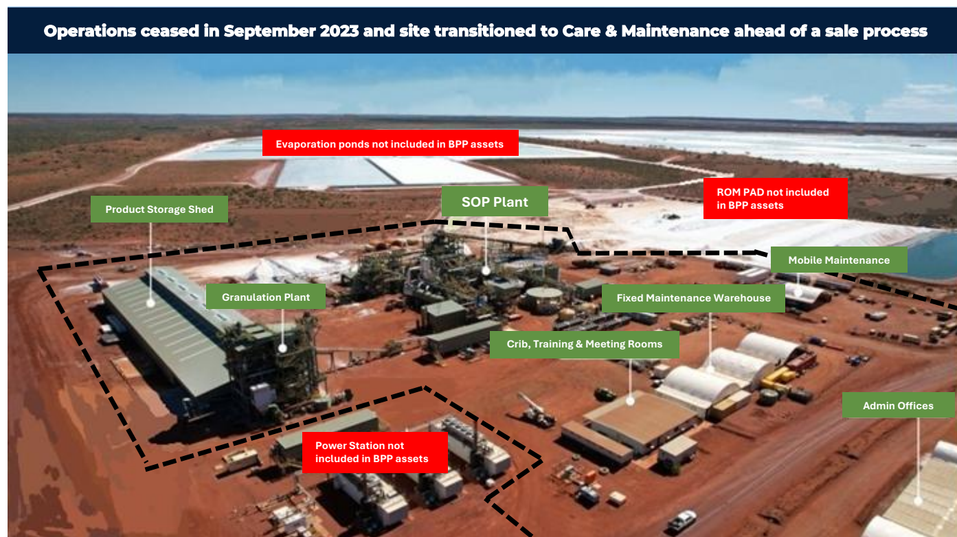
Figure 9 – Photograph of the Beyondie Potash Project in 2023 when in operation by Kalium. The assets include a fully constructed processing plant, site offices and maintenance infrastructure. Specific plant components include, KTMS crushing circuit, Kainite conversion circuit, column flotation circuit, liquor cooling heat exchangers, evaporative cooling circuit, product separation centrifuges, SOP recovery and granulation units, RO water plant and a bulk storage shed. 1
