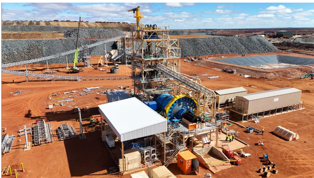
KGP Expansion Project nearing completion July 2026.
