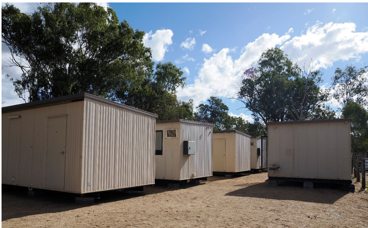
Figure 4. Four accommodation blocks in place next to kitchen/messing block. Covered walkways to be installed during commissioning.
