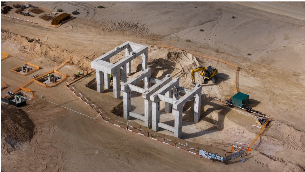
Figure 3: Concrete structures for the secondary and tertiary screening progressing towards completion.
