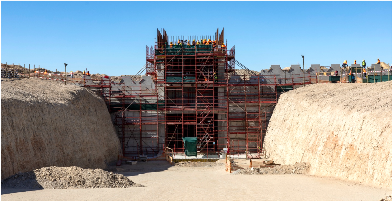
Figure 2: Below ground level view of the primary crusher building structure that has reached above ground level.
