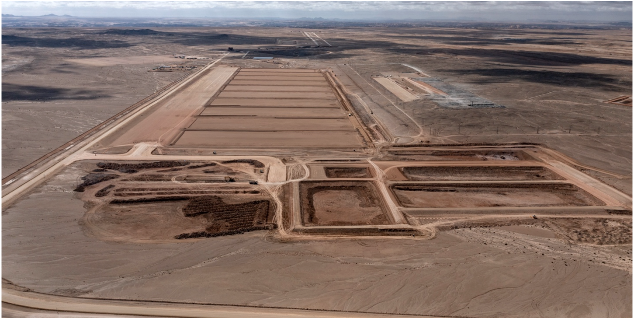
Figure 1: In addition to the heap leach pad earthworks, works have continued on the wet plant terraces and solution ponds.
