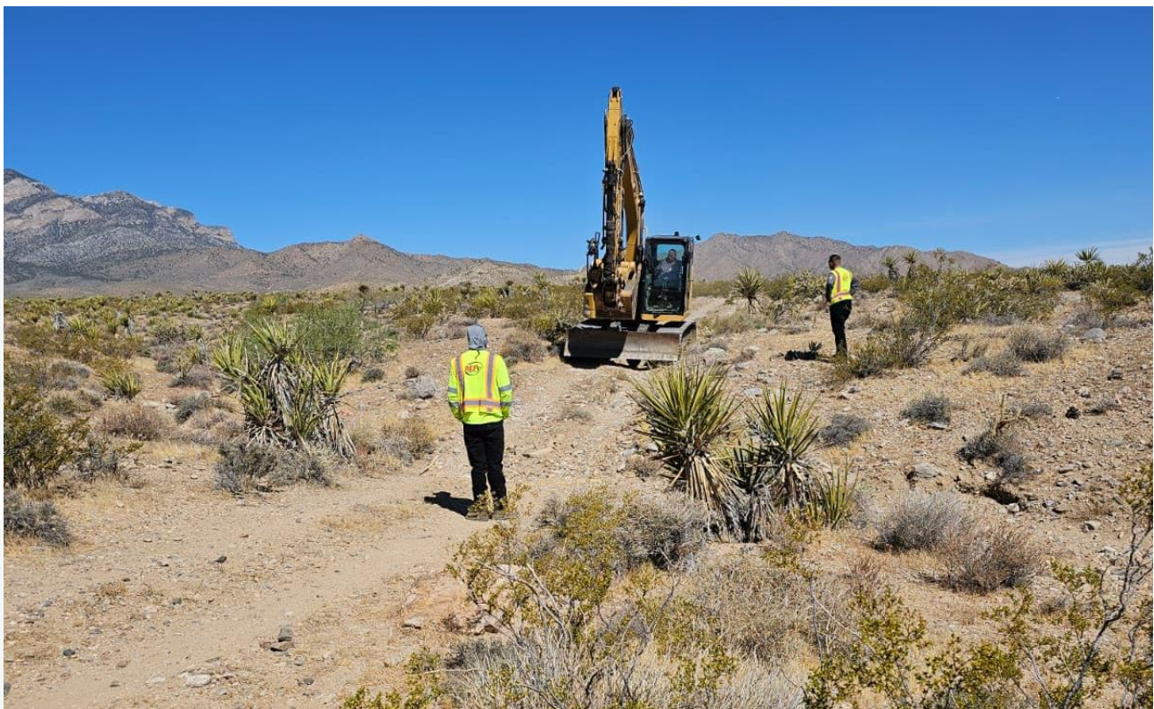
Figure 1: Access track upgrade works at Desert Star
