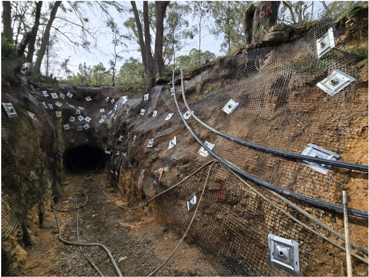
Figure 1: Photo of the current Sister Rose box-cut and portal looking North-East.
