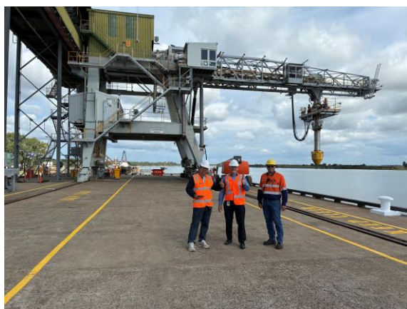
Figure 7: Sir Thomas Hiley Wharf, which supports dry bulk cargo at the Port of Bundaberg
