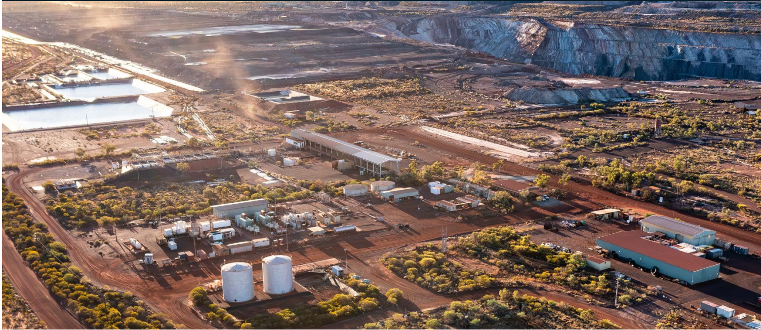
PARTIAL REFURBISHMENT OF SXEW PLANT: “B TRAIN” TO SUPPORT ~6,000 TPA PRODUCTION 2
