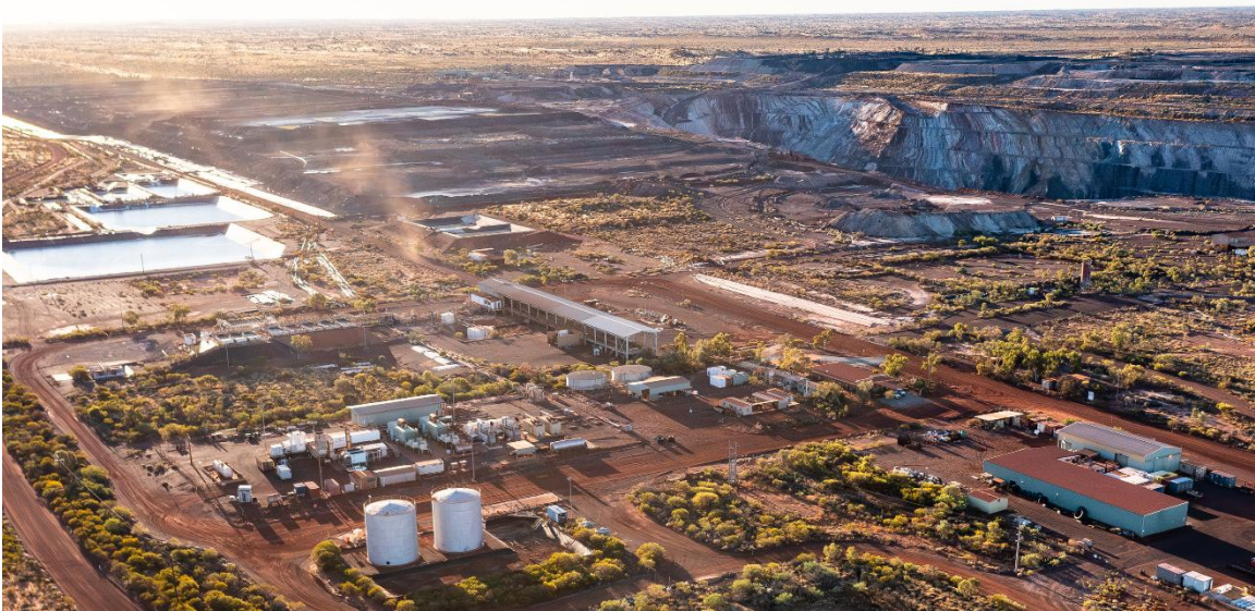
25,000 TONNE CAPACITY SXEW PLANT
