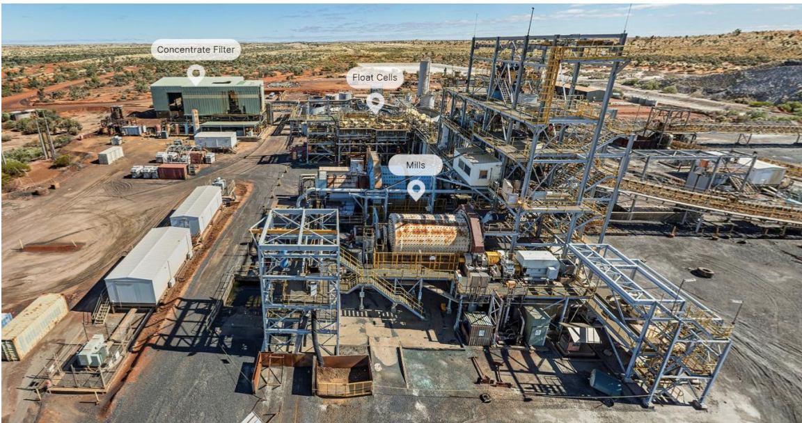
50,000 TONNE FLOAT PLANT, 2.8 MTPA MILL
