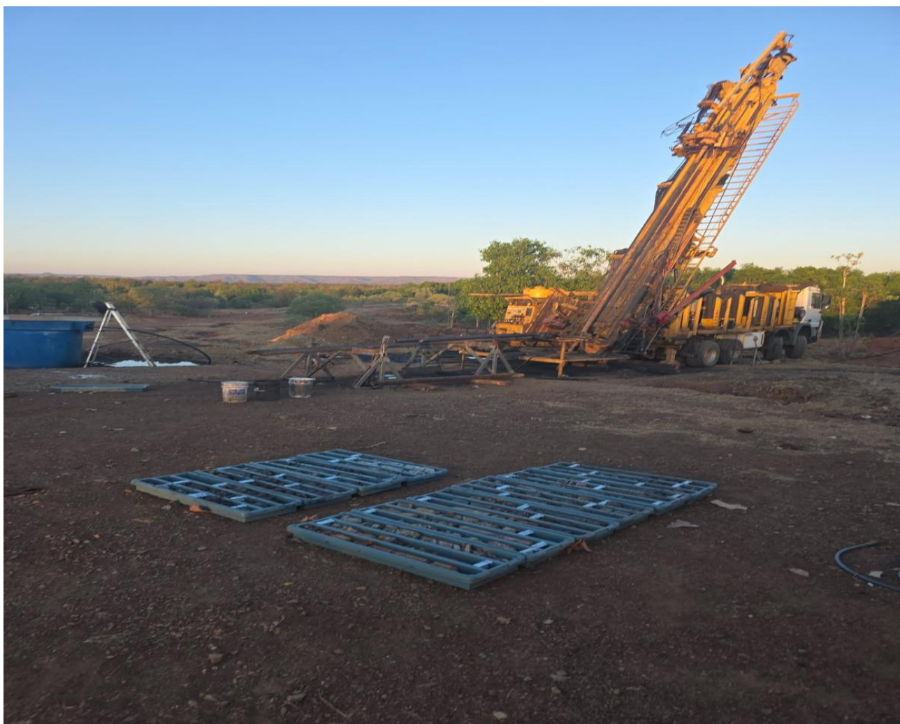
Figure 1: Drill rig on site at Bridge Creek
