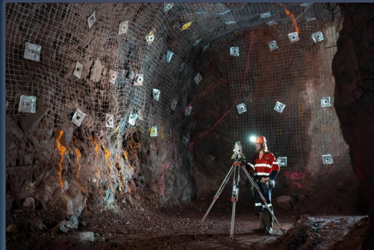
Established underground development
