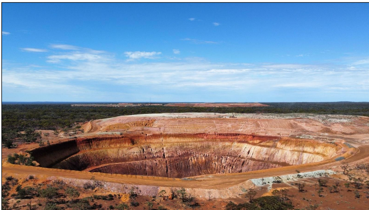
Figure 1 - Eureka open pit, aerial view looking east. Note the excellent wall condition
