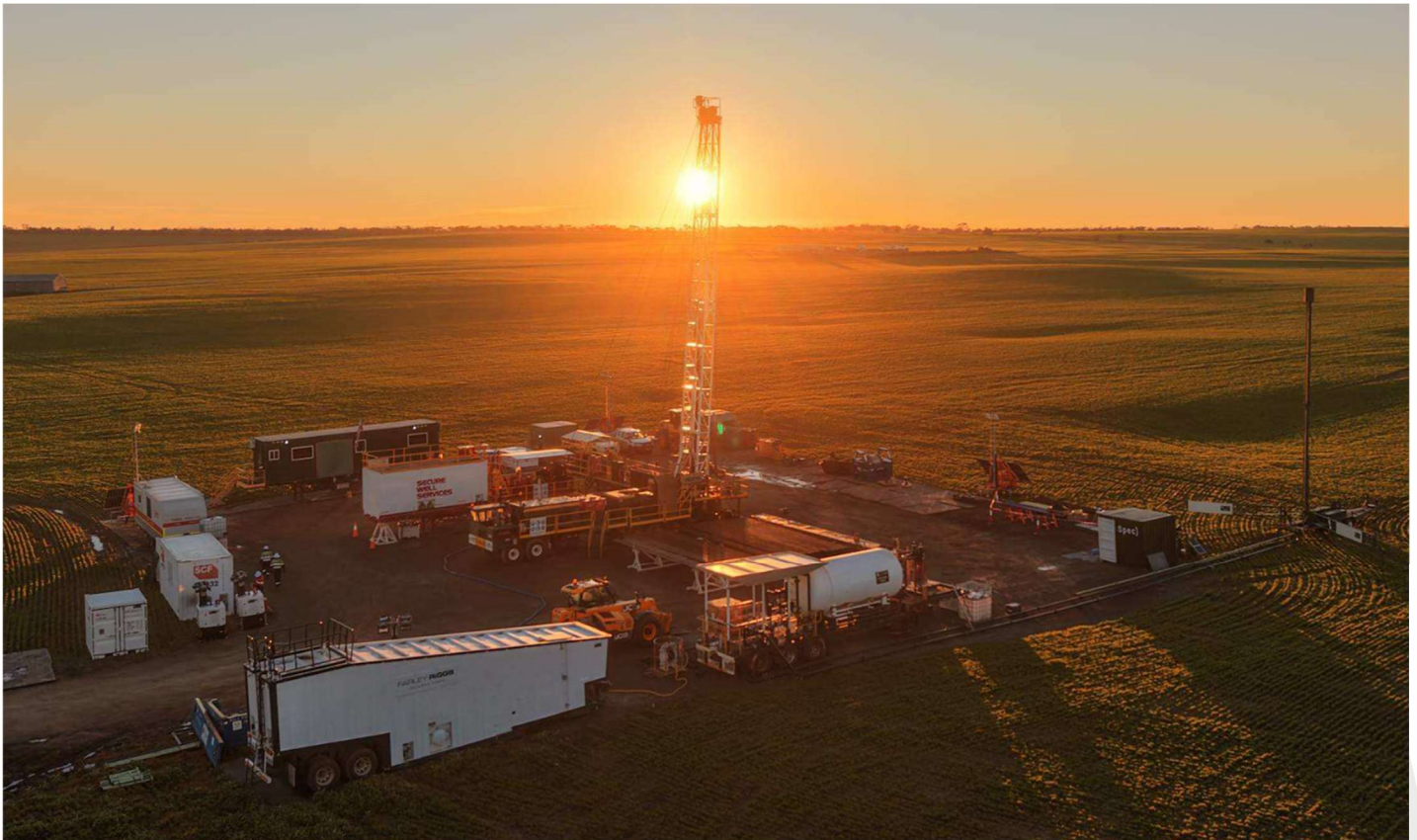
SWS Rig 04 onsite at Ramsay 1 and preparing for flow testing
