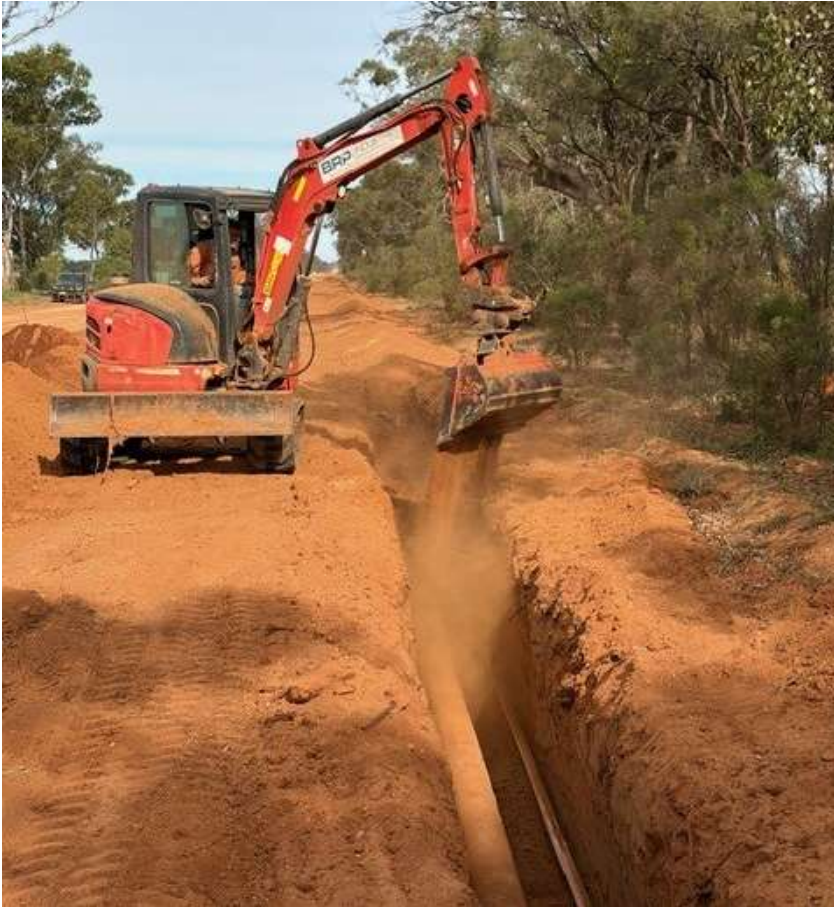
Figure 1: Trenching activities on the services corridor
