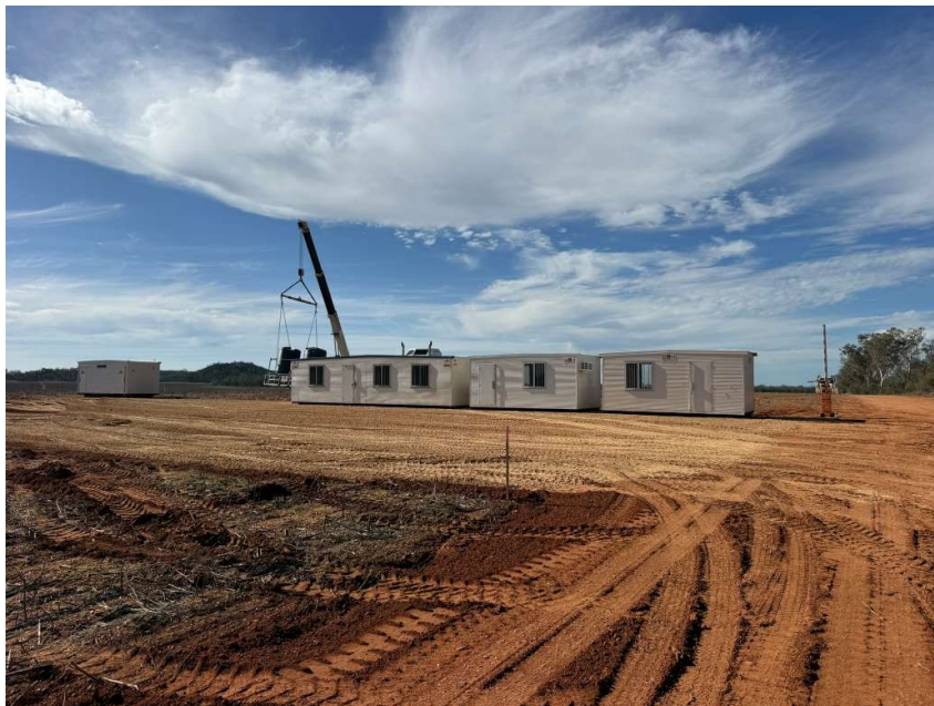
Figure 3: Site office construction
