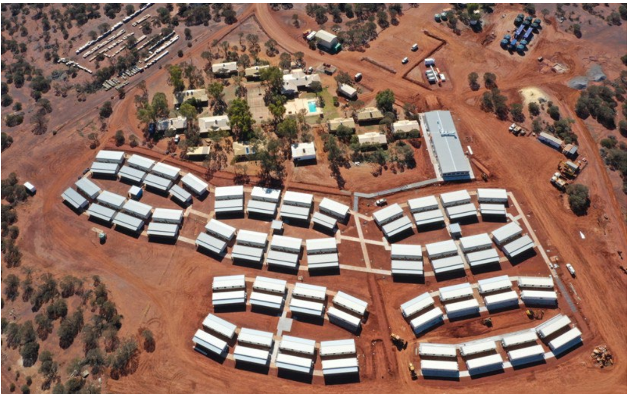
Figure 12 – Camp and expansion works
