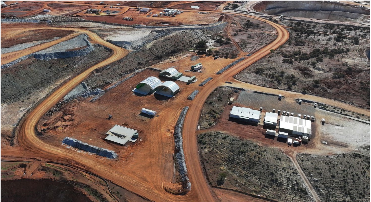
Figure 11 – Mining office and contractor workshops nearing completion
