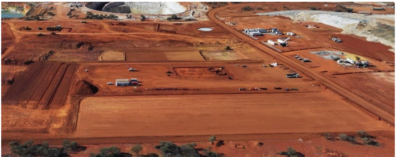
Figure 6 – Youanmi Processing Plant earthworks and civil works
