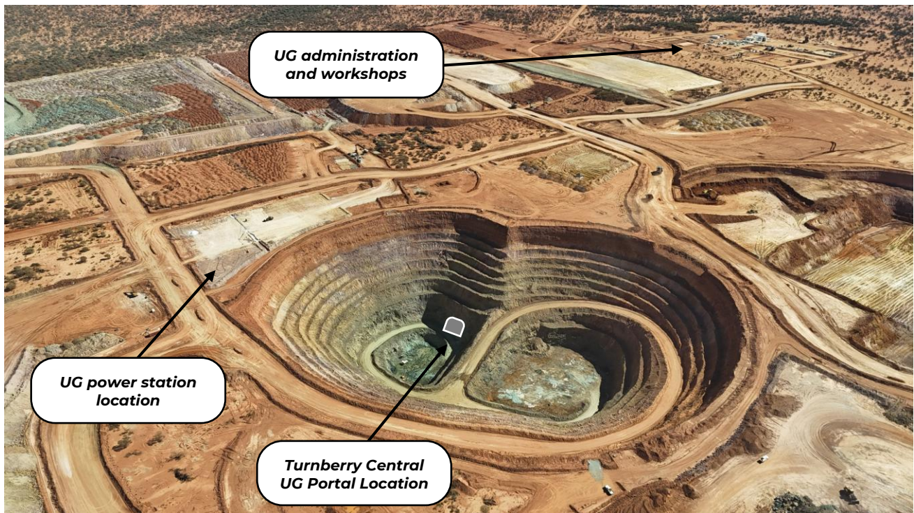
Figure 3: Turnberry Central pit showing the location of the first underground portal on the western side of the pit, the power station location, administration area and workshops (June 2026).
