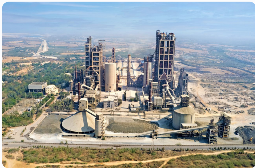
Ambuja Cements' Sanghi cement plant in Sanghipuram, Gujarat's Kutch district
