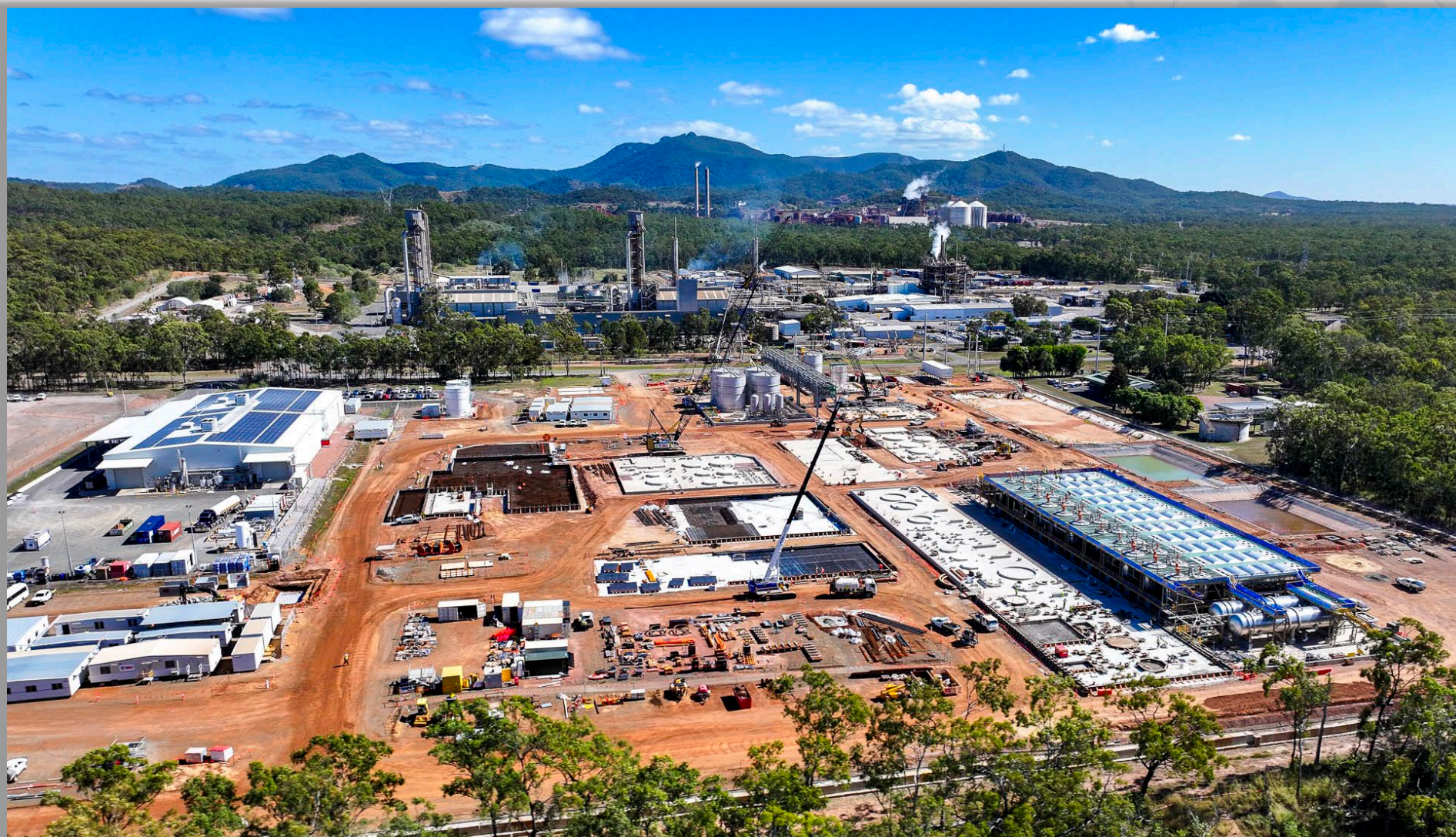
Stage 2 construction – looking west.
