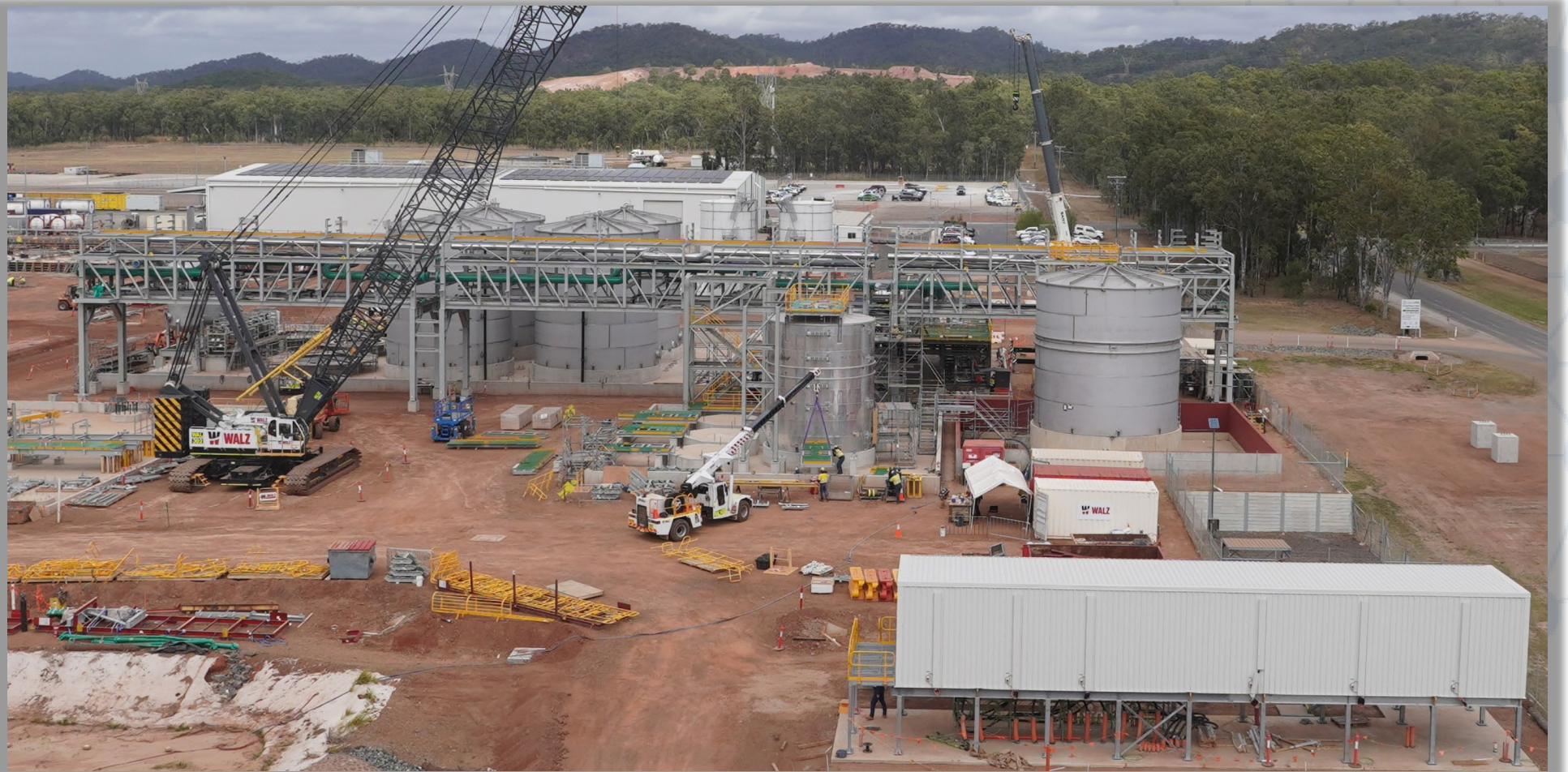
Stage 2 Construction - First three pipe rack and substation – Looking South
