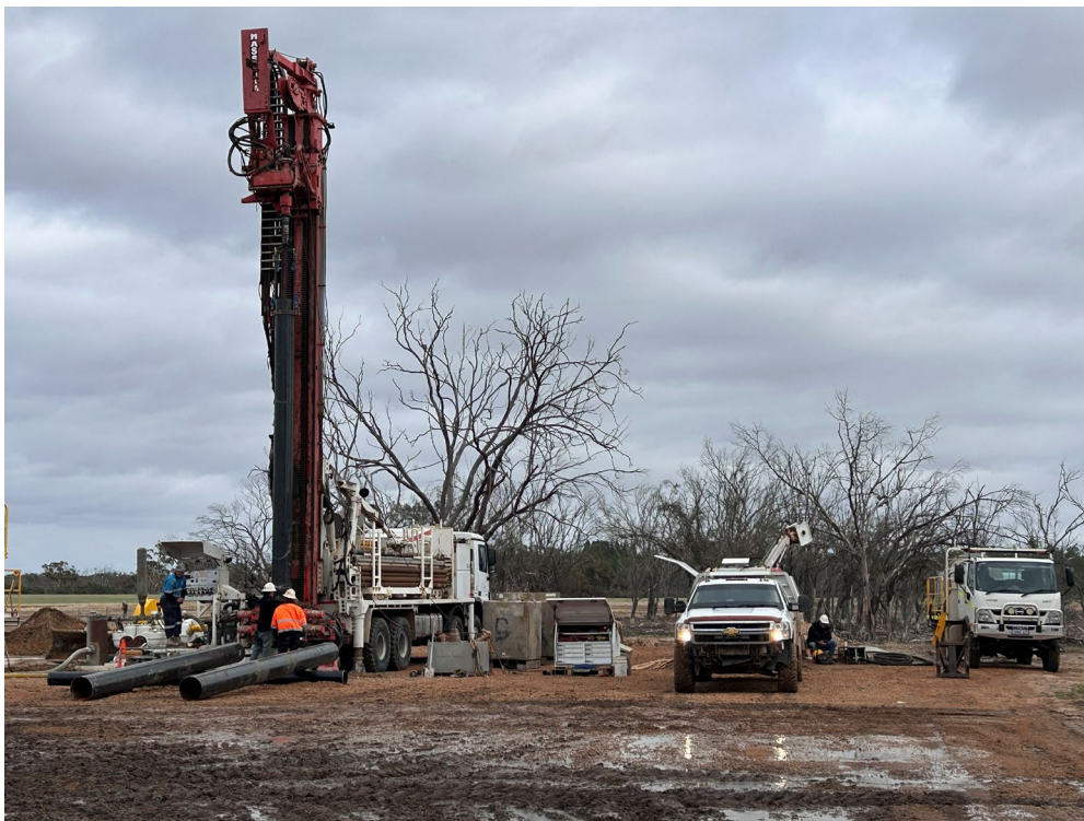
Water bore drilling and bore development at the Gillingarra borefield 2026 programme.
