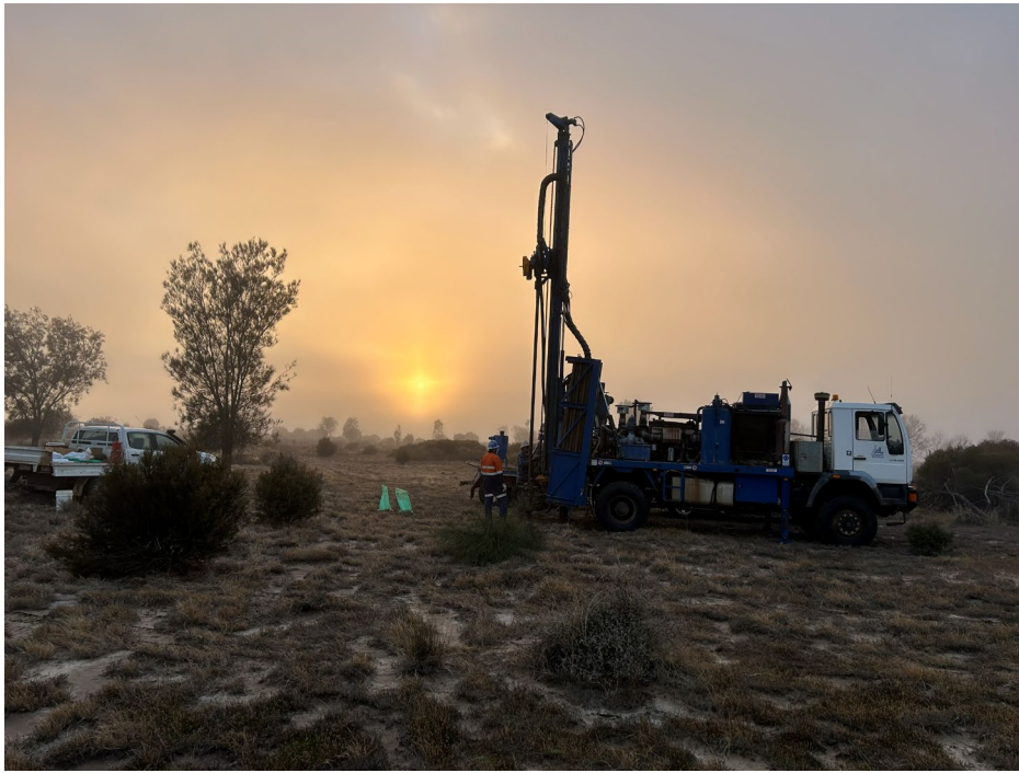
Aircore drilling within the proposed tailings management facility footprint.
