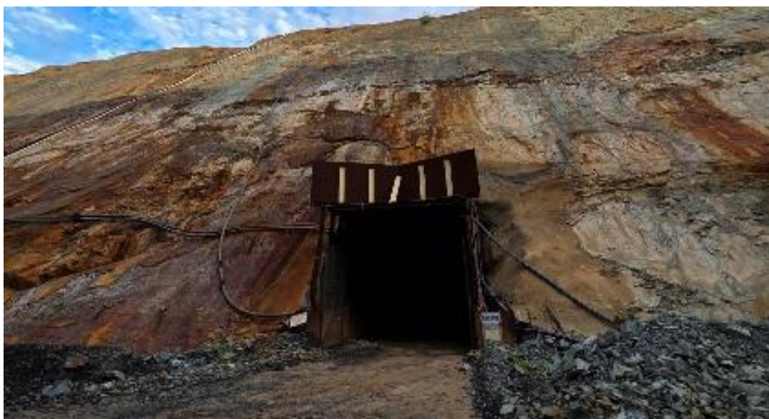
Figure 1: Photo of the Comet Portal, with gates open for underground access
