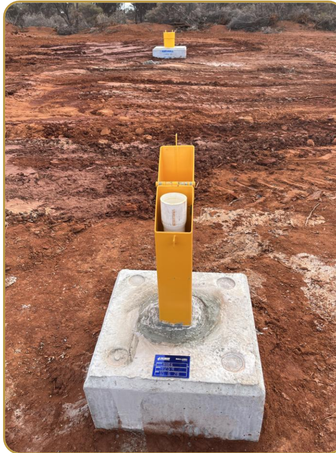
Production bore background and monitoring bore foreground
