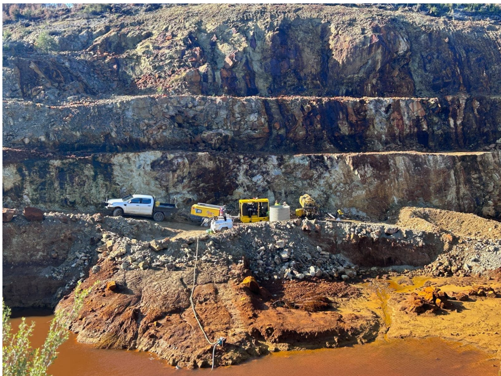
Figure 14 Granville East pit
