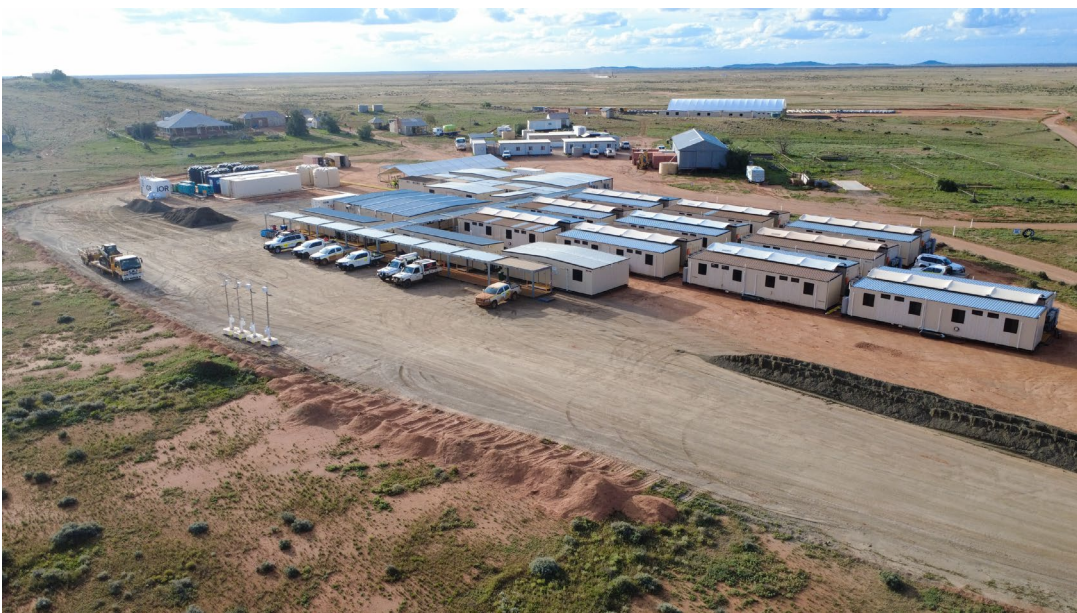
Figure 4 Sandfire’s recently completed 80 bed onsite camp located adjacent to Kalkaroo homestead and Havilah’s long term exploration camp. The new core processing facility is under construction (white roof in the middle distance).
