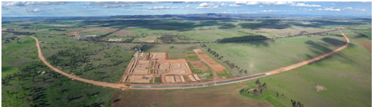
Newell Highway works looking east.
