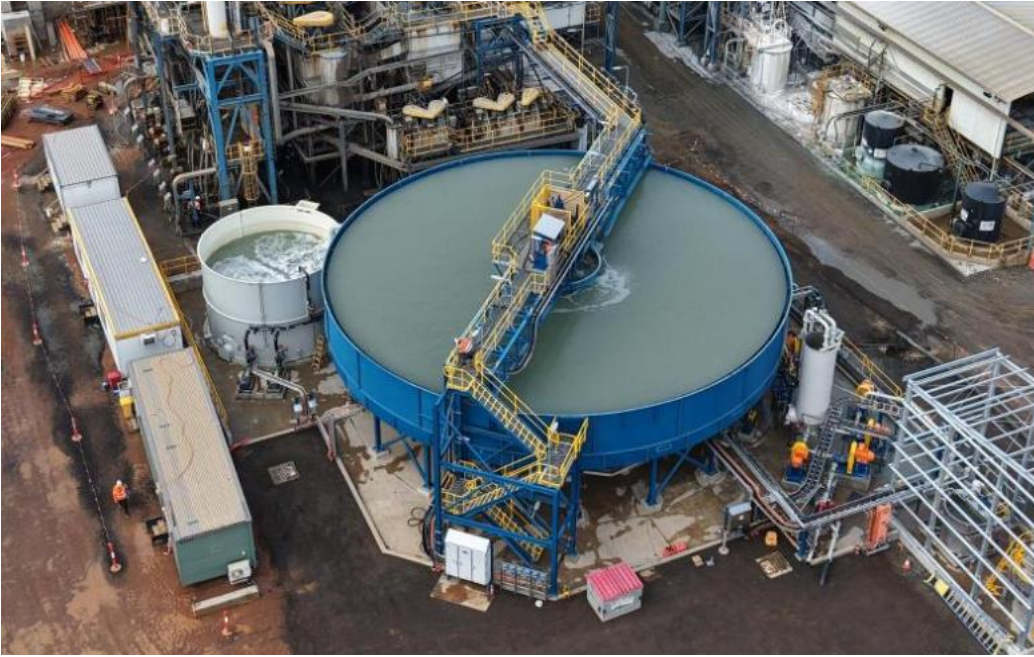
Photo: New 22m tailings thickener now in operation at Peak (June 2026)
