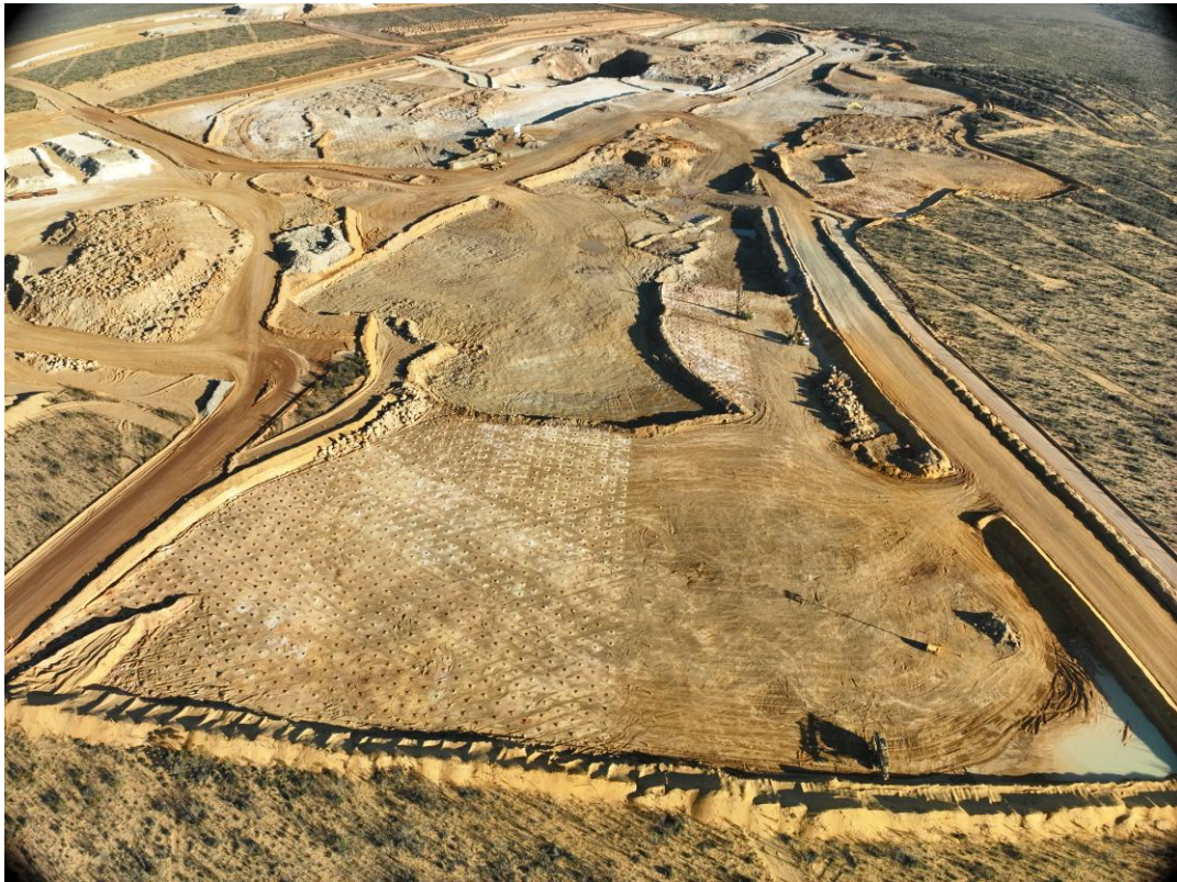
Figure 4: General View of Mining Activities 15 July 2026
