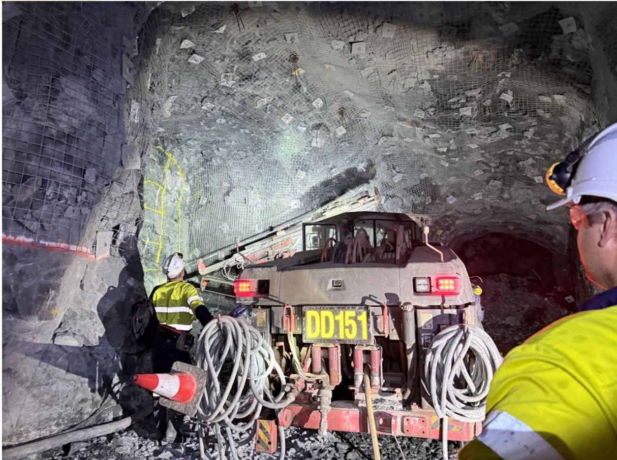
Figure 2: Underground development activities at CMA
