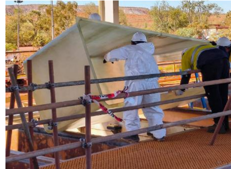
Installing fiberglass inserts for EW cells
