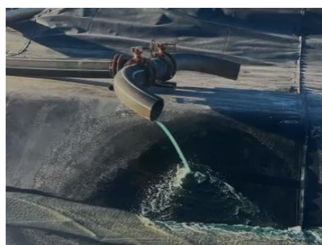
Off-flow piping discharging copper rich solution
