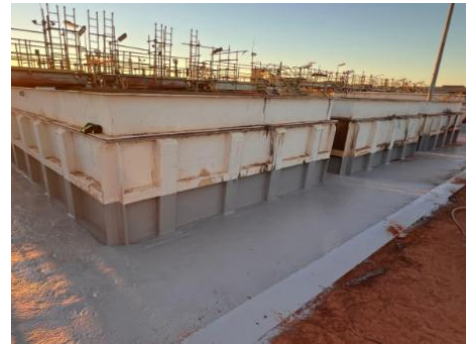
Acid proofing at mixer settlers complete
