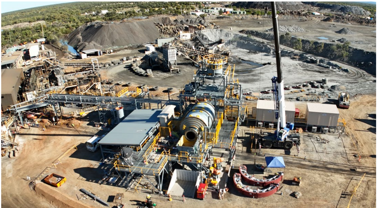
Photo 2: Construction progress – grinding area.
