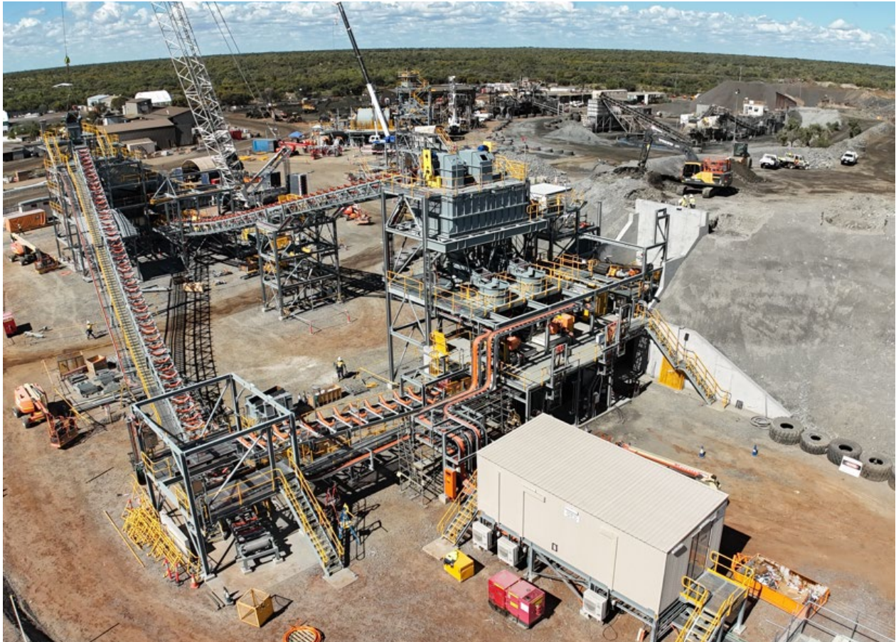
Photo 1: Construction progress - crusher and screening areas.
