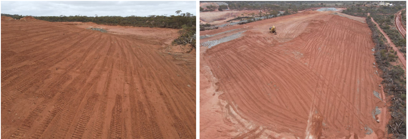
Figure 2: Rehabilitation of the waste dumps continues with deployment of topsoil stockpiles in parallel to the mining operation.
