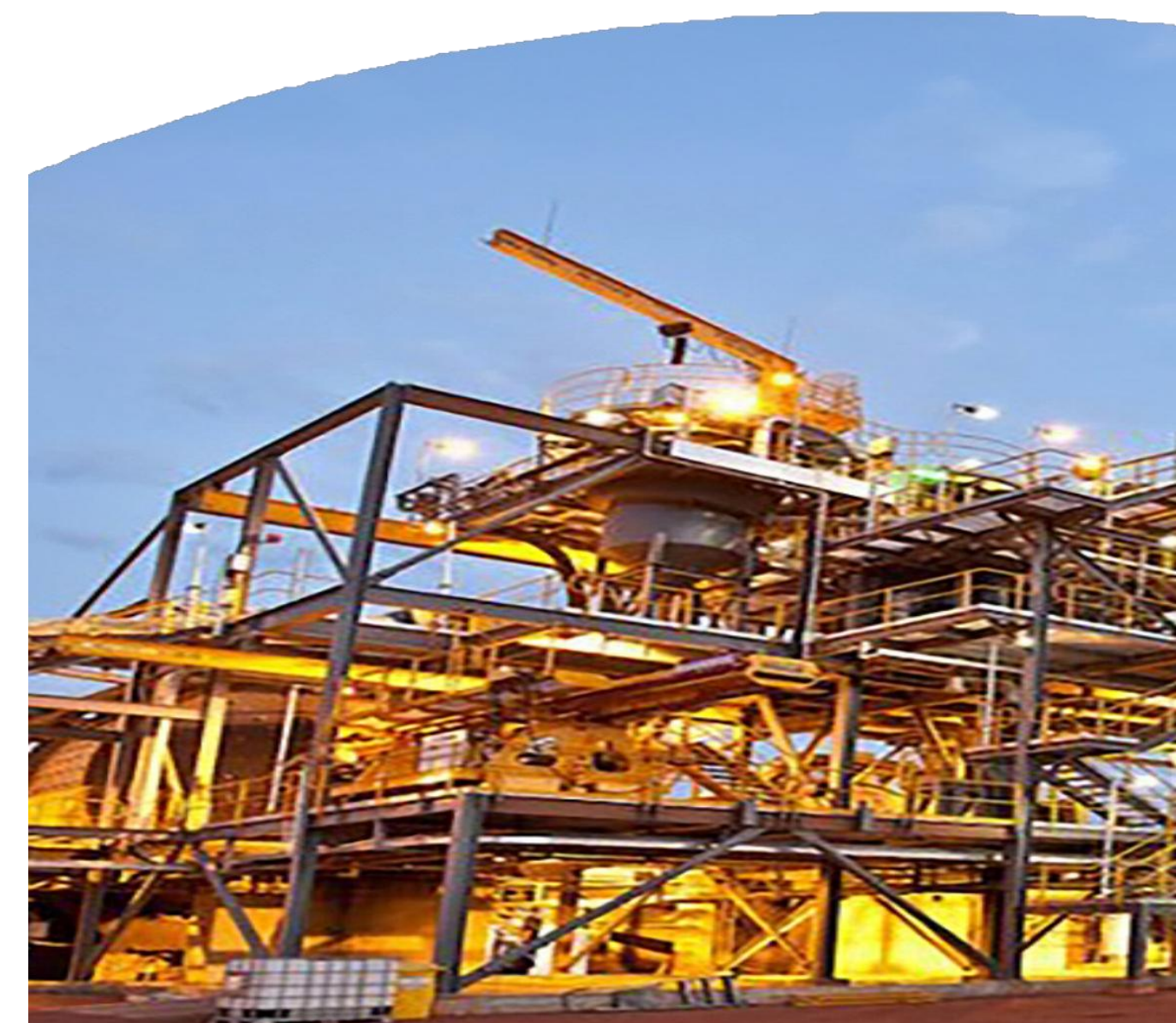
DeGrussa Processing Plant
