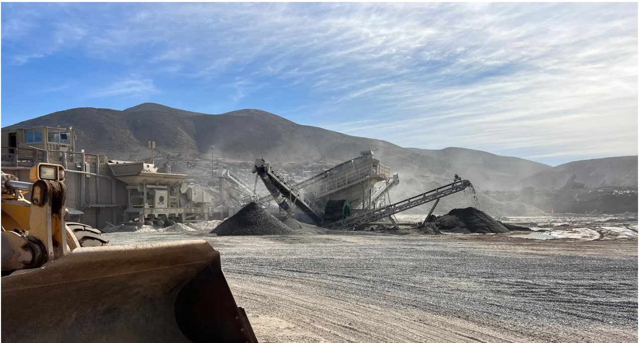
Image 1: Islon plant in operation with added conveyors and washing unit
