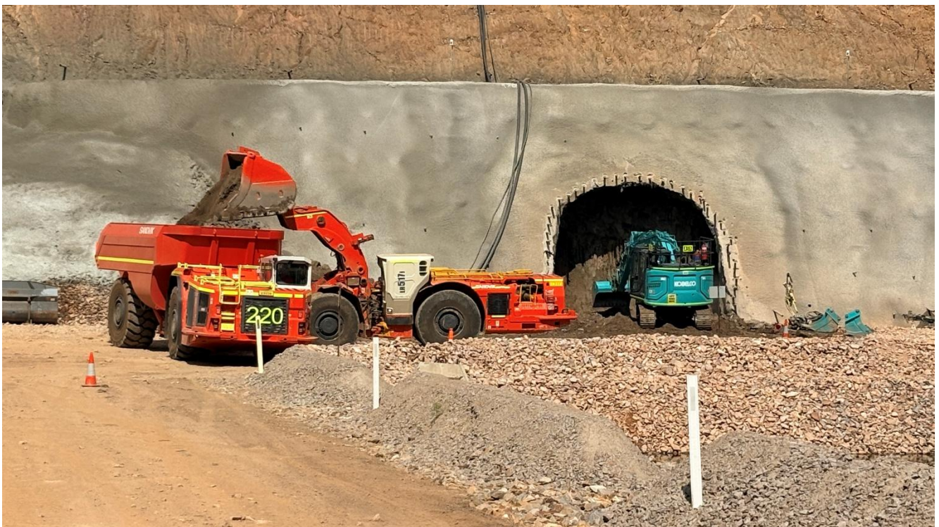
Figure 2 BP33 underground decline progress
