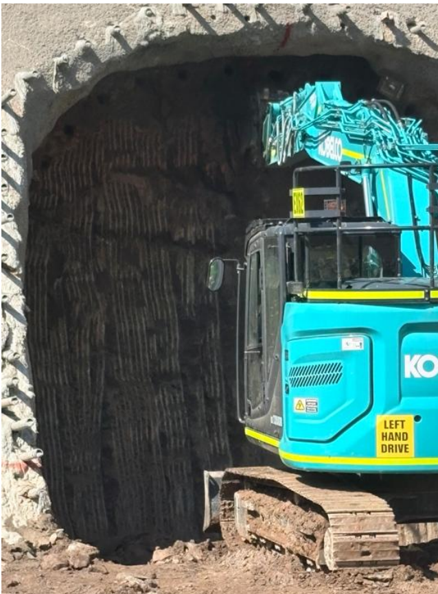
Figure 4 BP33 portal cut progress
