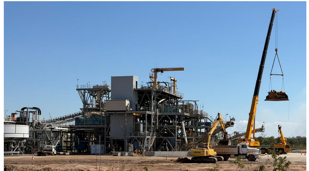
Finniss DMS plant (top). Secondary DMS screen lifted out for refurbishment upgrade (bottom)
