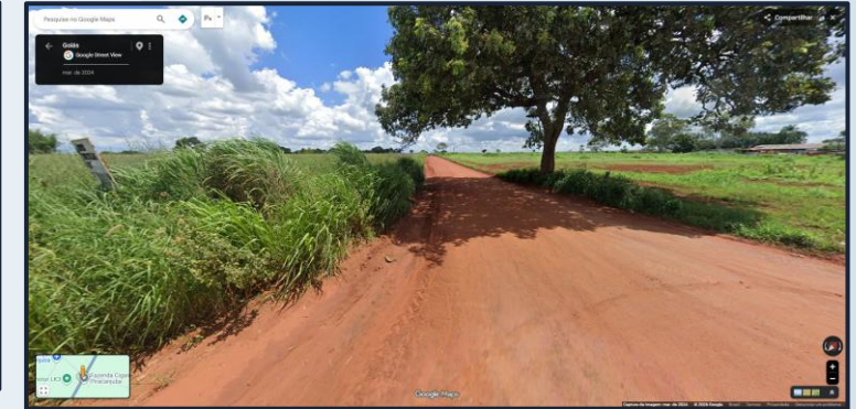
Section of unpaved local road near Piracanjuba. Source: Google Maps – Street View (2024).
