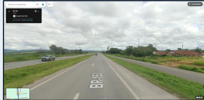
Condition of State Highway BR-153 (Belém-Brasília Highway), the main connection corridor between the region and the state capital, Goiânia. Source: Google Maps – Street View (2025).
