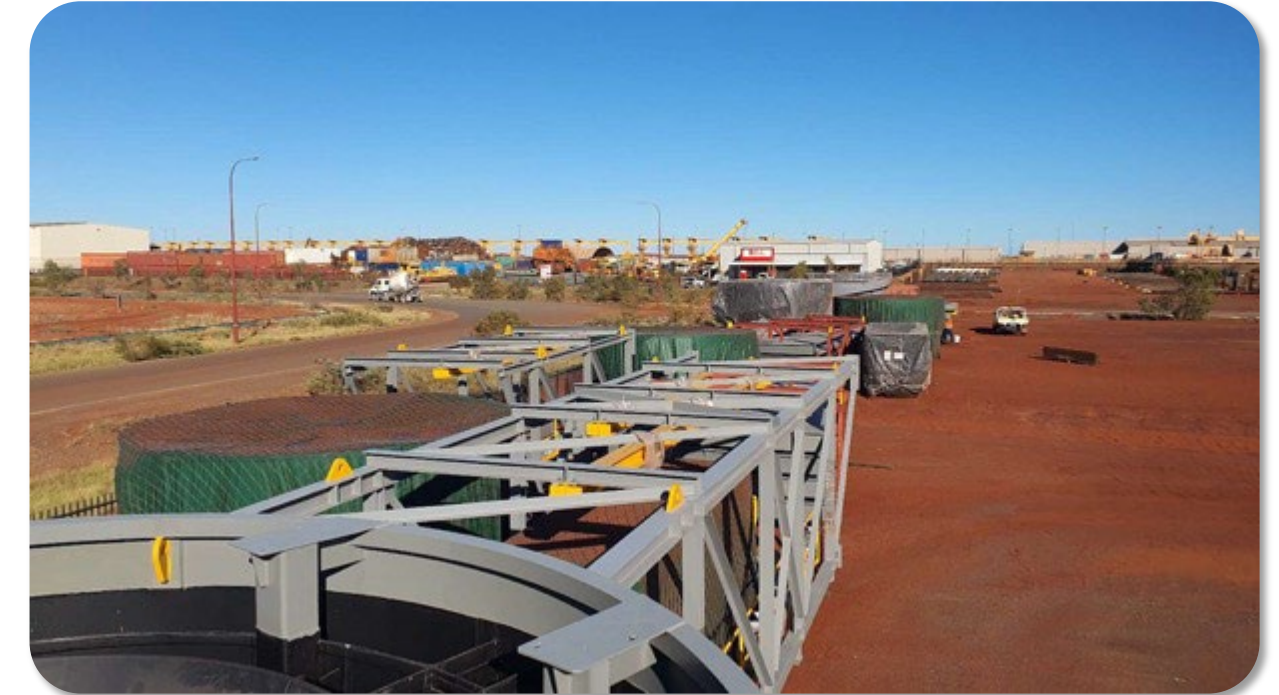
Flotation Cells & Structural Steel ready for installation.
