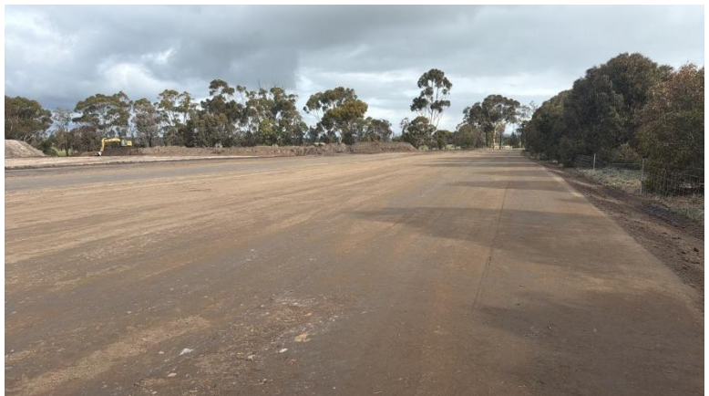
Workforce Accommodation Village site preparation well underway.
