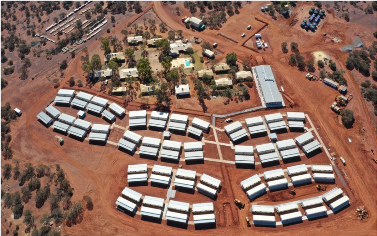
Figure 11 – Camp works nearing completion
