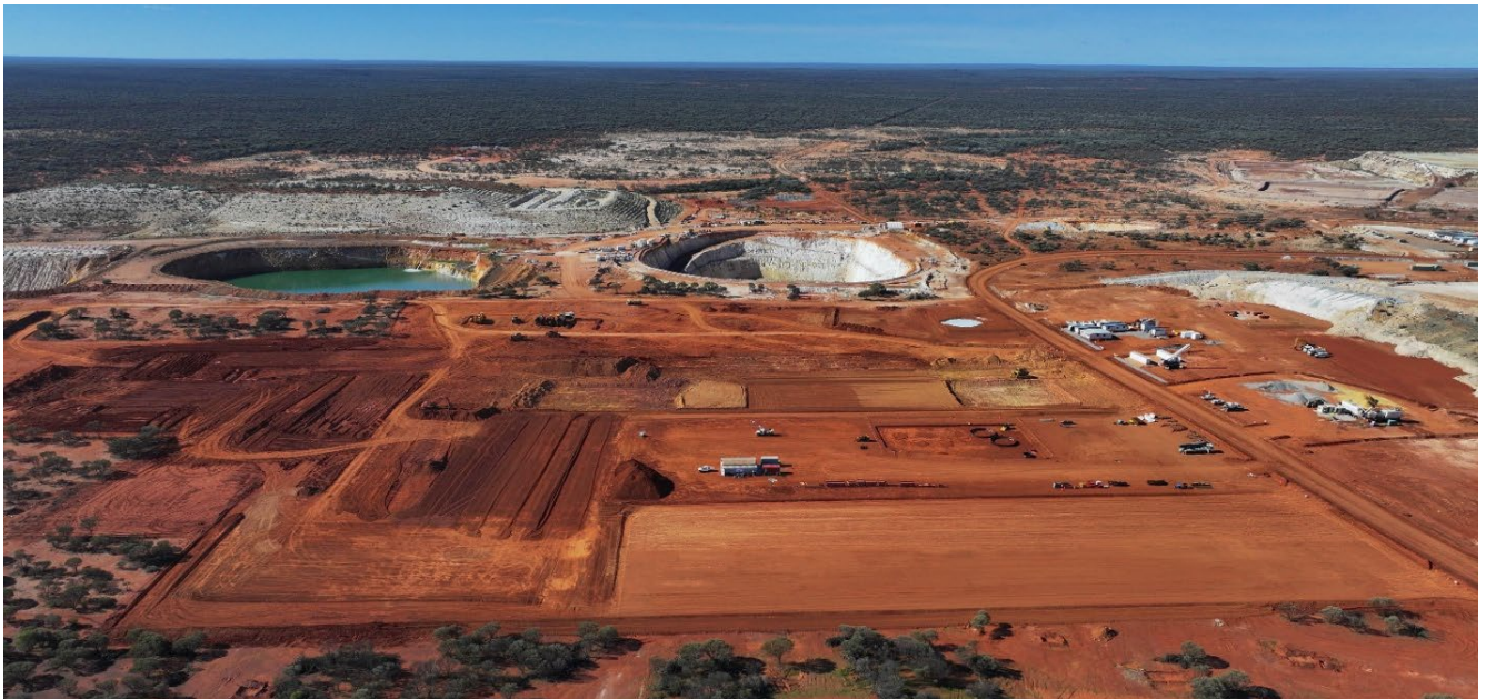
Figure 1 – Site set-up and civil works underway – looking East
