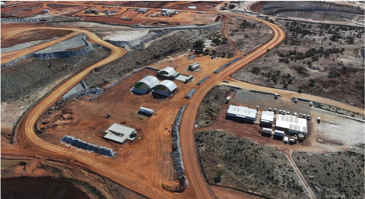
Figure 10 – Mining offices, changerooms, workshop and wash bay
