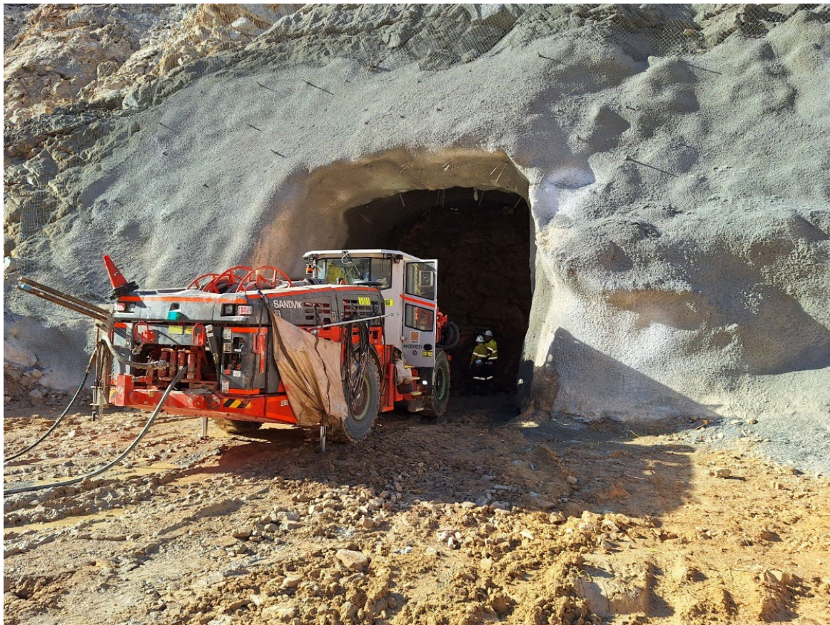
Figure 7 – Pollard Decline mining underway
