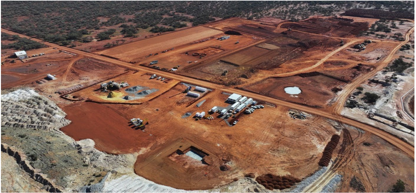
Figure 2 – Site set-up and civil works underway – looking North-West
