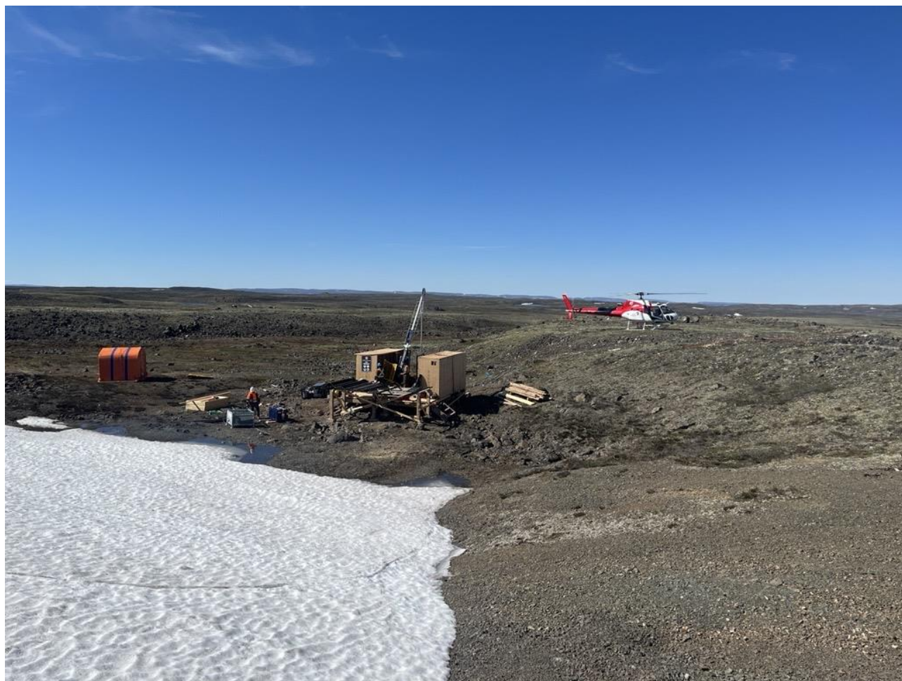
Figure 7 - Diamond Rig at Drill hole DAN26026.
