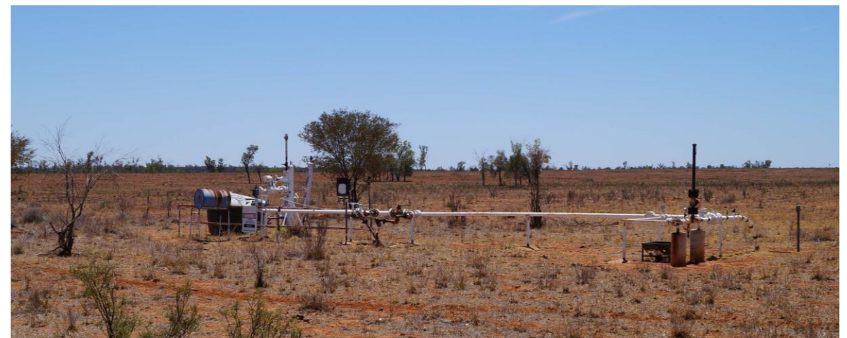
Major-4 production well and gathering system
