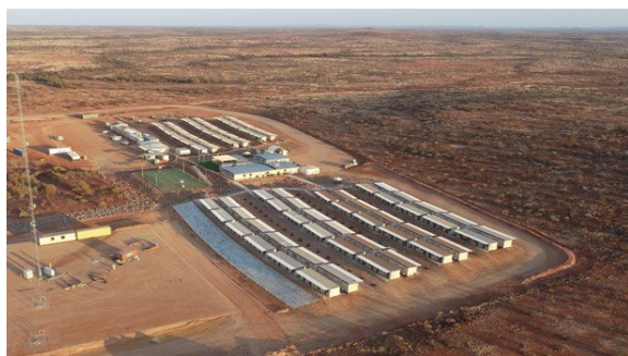
Figure 4: Kurrbili Accommodation Village
