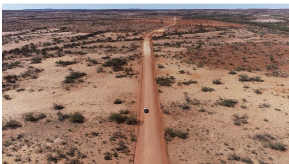
Figure 6: Site access Road Construction
