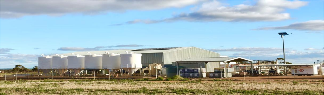
Fig 1. Wubin facility expansion project (June 2026)
