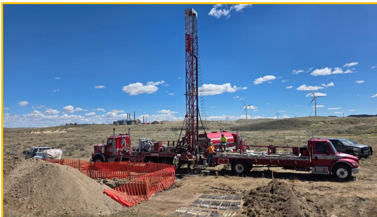
FIGURE 4: MUD ROTARY DRILL RIG AT MINE UNIT 2
