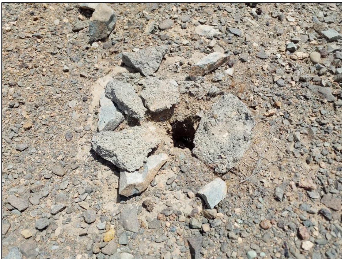
Figure 4.2: Some drill collars at Daris East have been vandalised, with building materials and metals removed
