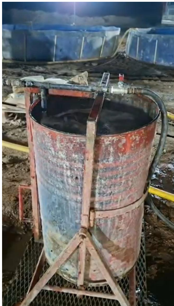
Figure 6. Brine being pumped from 110m using airlift on rig for packer test of sample from that 5m interval.
